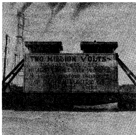
At left, the “lightning” formed a lace-like filament in an 830,000-volt sustained arc-over during a test of a huge Boulder Dam disconnect switch at Ryan. Above, a sign brags about “the highest voltage ever produced,” in another test at the Lab.
