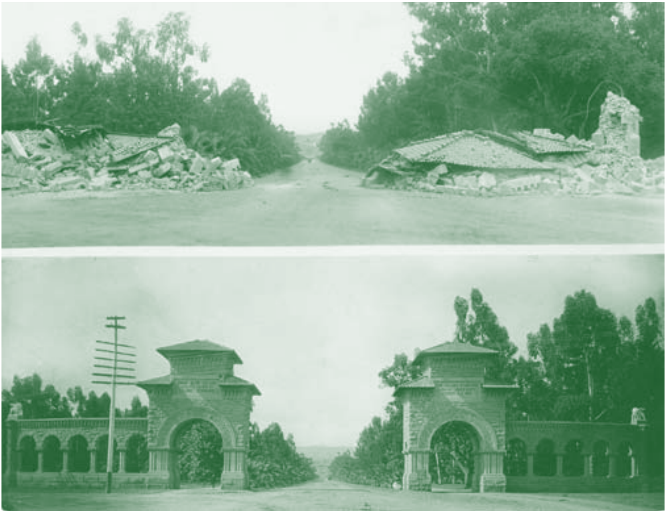
The university's entrance gates at Palm Drive and El Camino Real collapsed into piles of rubble.
