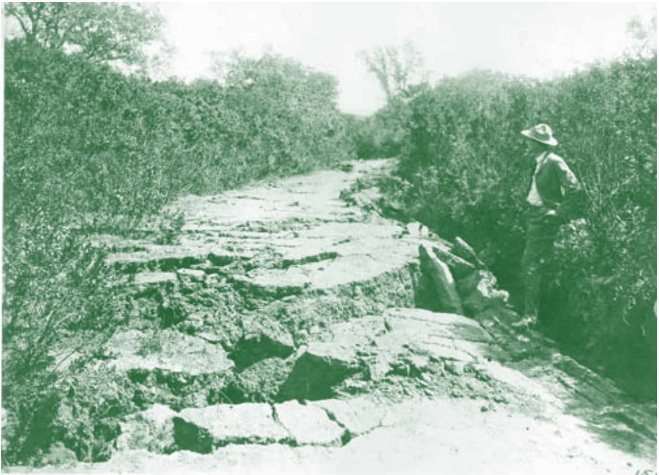
The quake caused the earth to buckle along the fault line on Alpine Road, to the west of campus.
