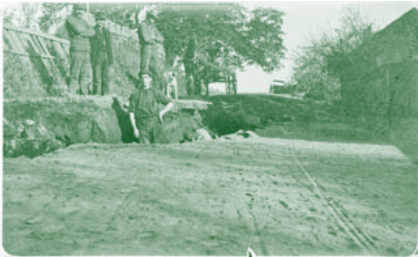
An hour after the earthquake, San Jose photographer F. E. Caton took this picture of a caved-in roadway in the Santa Cruz mountains.
