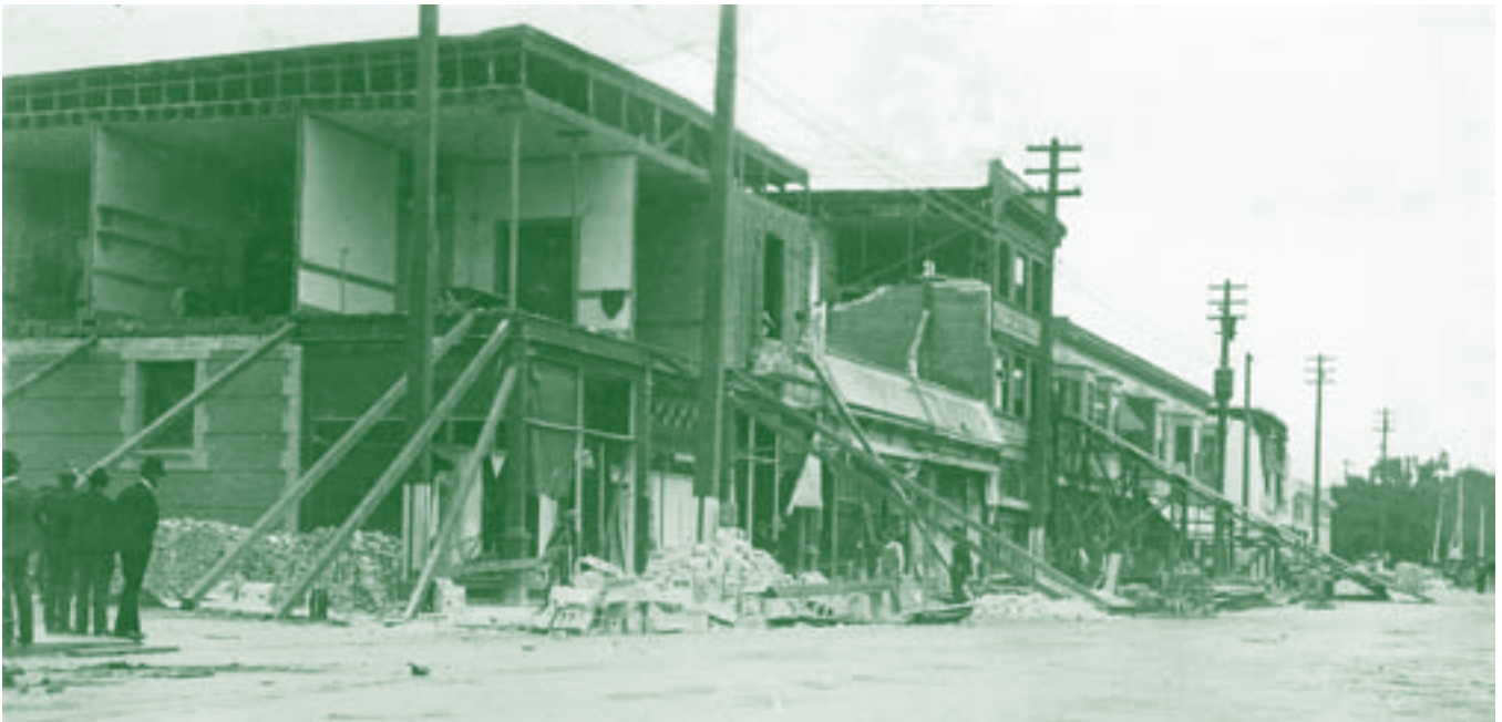
Timbers brace quake-damaged buildings at University Avenue and Emerson Street in Palo Alto.
