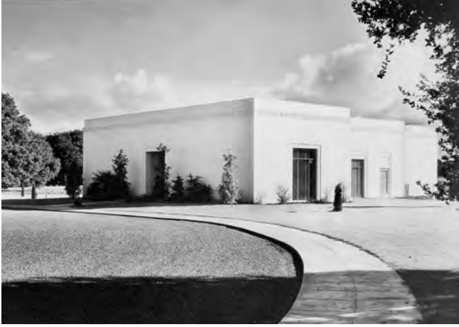
FIG. 3: This Art Deco mausoleum in Palo Alto's Alta Mesa Memorial Park, designed by Birge and David Clark and built in 1933, reflected contemporary architectural trends.
